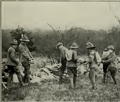
"GOOD TURN." Scouts repairing a stone wall.
